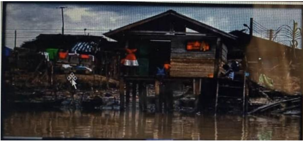
PICTURE 2: SHOWING RESIDENTIAL HOUSES BUILT ON TOP OF POLLUTED WATER
