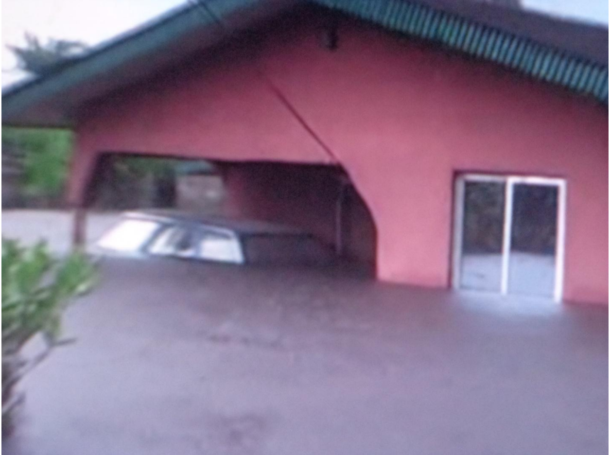
Fig. 3: One of the many houses and cars ravaged by the uncontrollable flood in Agadama community.
