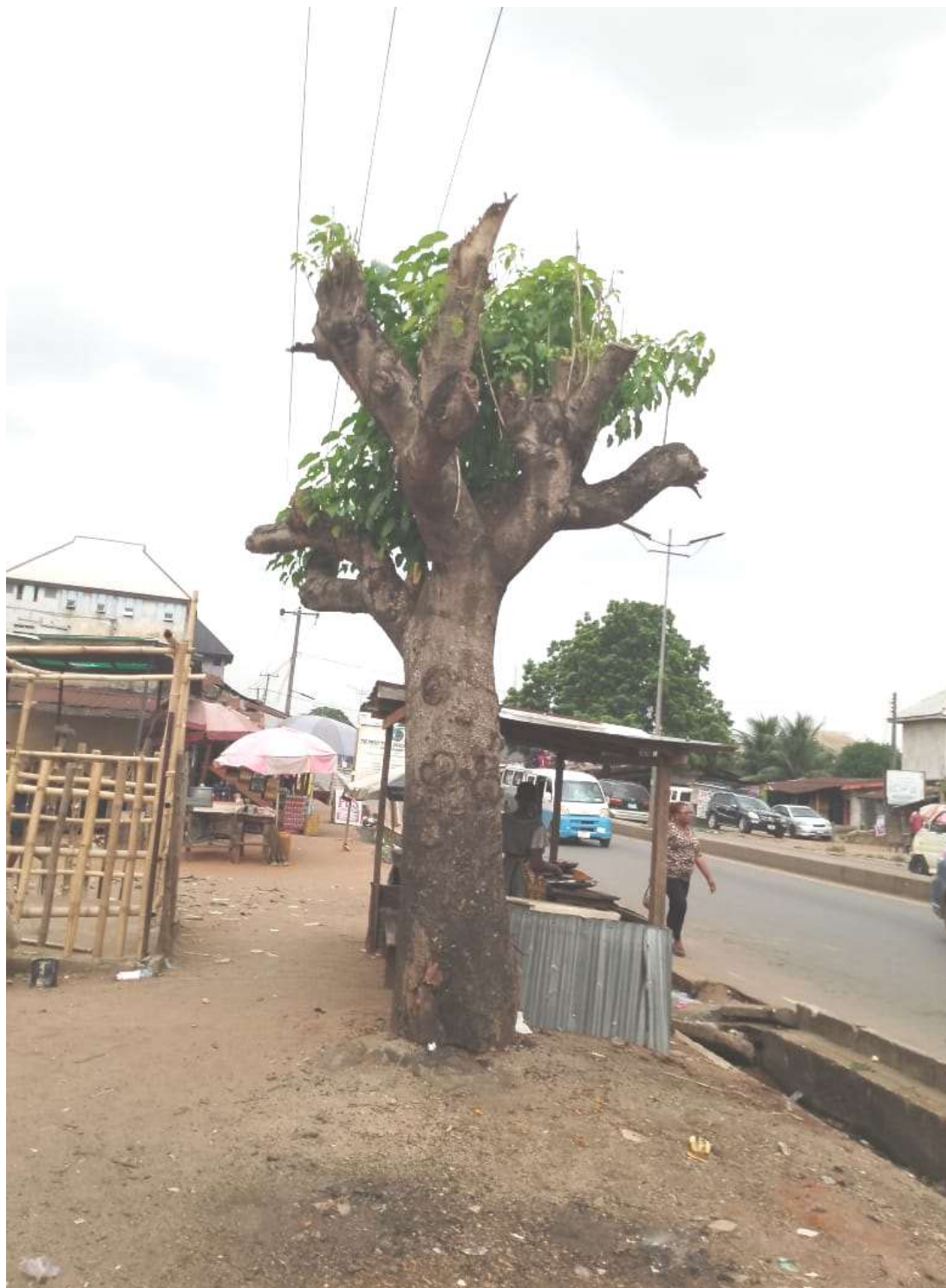
Plate 3: Heavily pruned tree under the High tension electric cable
